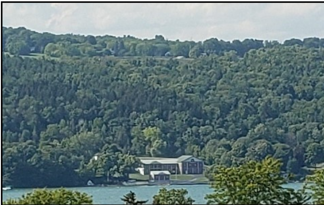
Water Treatment Plant, 1515 West Lake Rd., Penn Yan,
